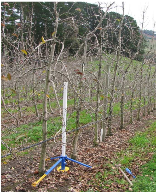
IMAGE 7. INSTALLING ACCESS TUBE
